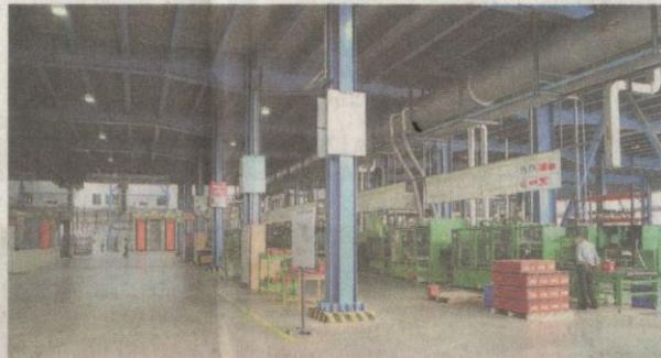
Exide's punched grid battery manufacturing unit in Haldia, Bengal
